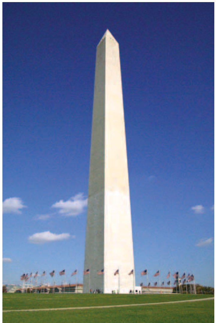
American citizens were first energized to build the Washington Monument during the centennial of Washington's birth. Photo courtesy of the National Park Service.
